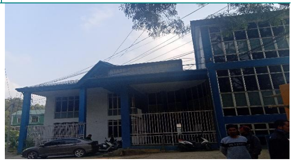
SITE PHOTOS – BUILDING OF LIBRARY
