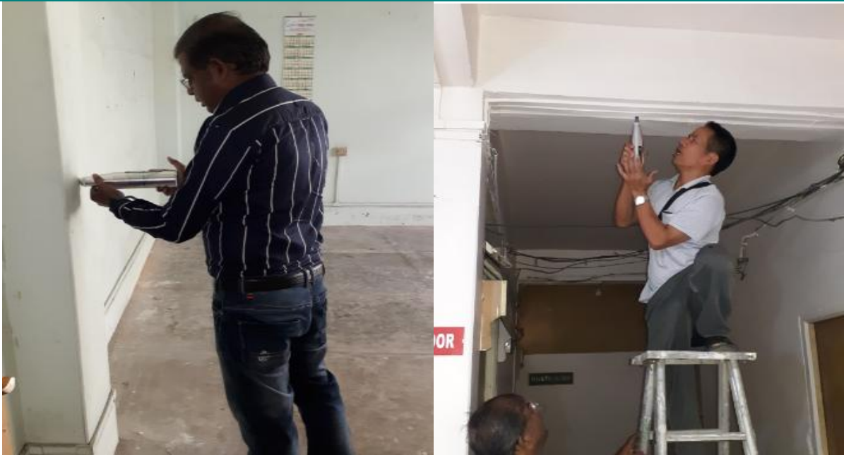
FIGURE 1-11: PHOTO SHOWING OPERATION OF REBOUND HAMMER
