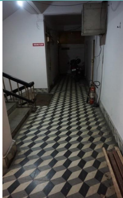
FIGURE 1-7: IMAGE SHOWING EXISTING STAIRCASE CONDITION
