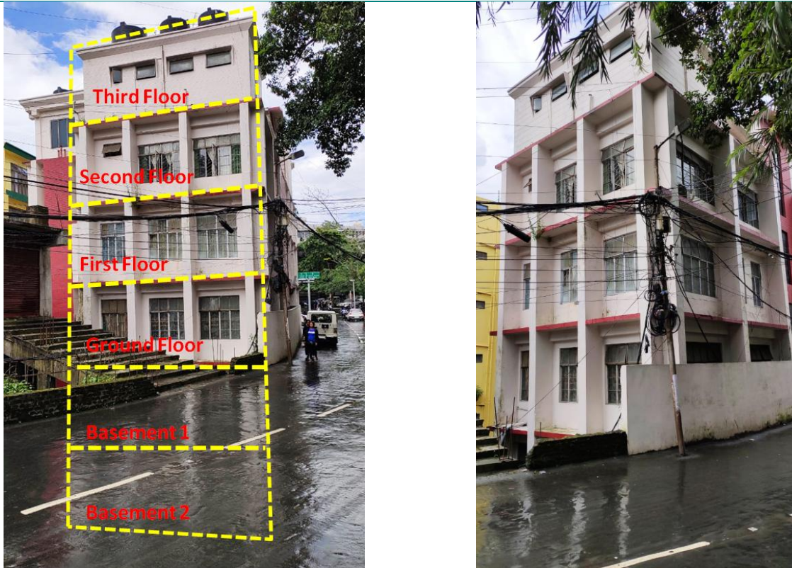
FIGURE 1-3: IMAGES SHOWING EXISTING SIDE FACADE
