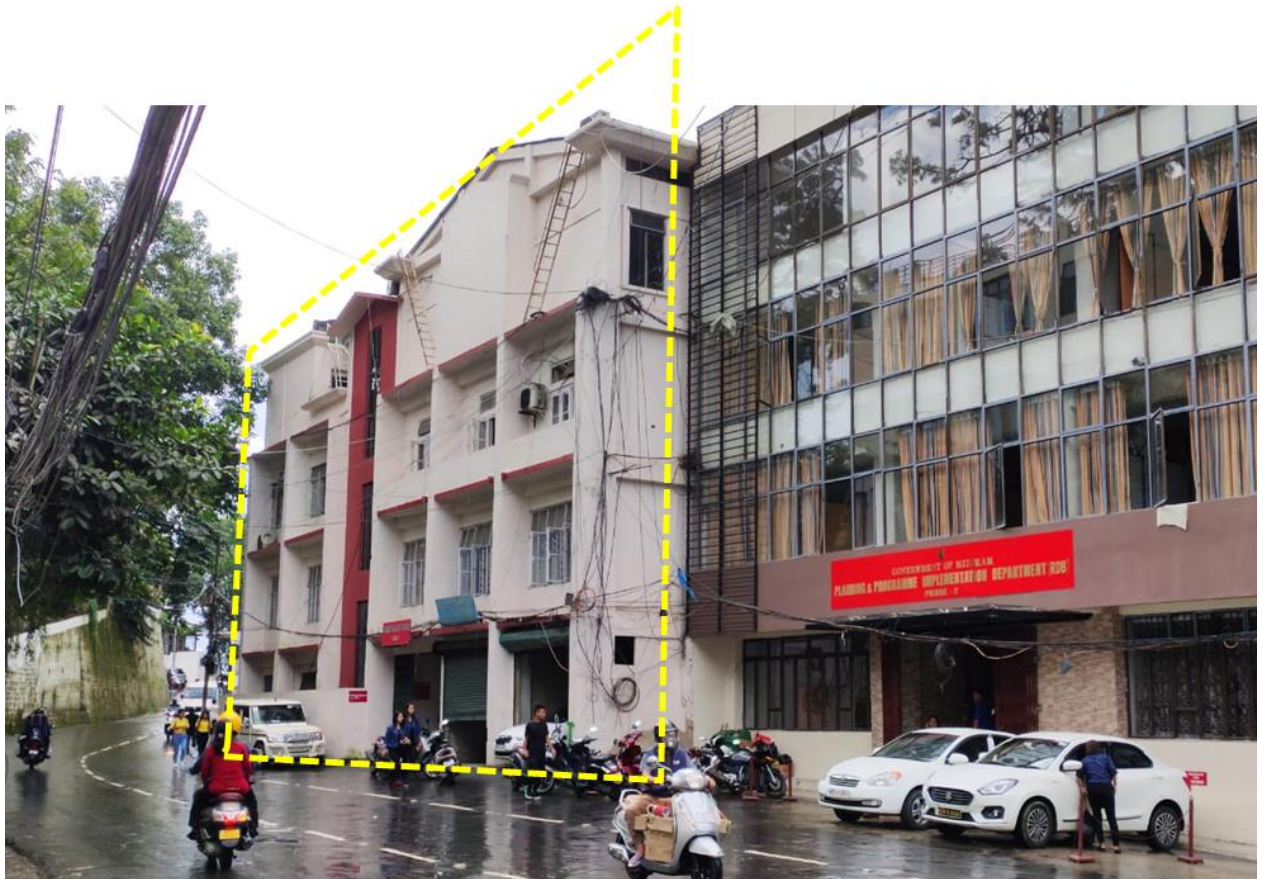
FIGURE 1-2: IMAGE SHOWING EXISTING FRONT FACADE
