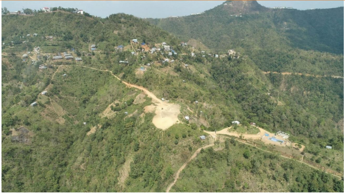
Figure 13: Lack of proper access road to site.
